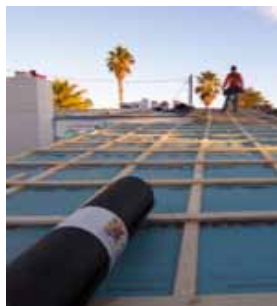
Fig. 13: Decked roof with vent space
