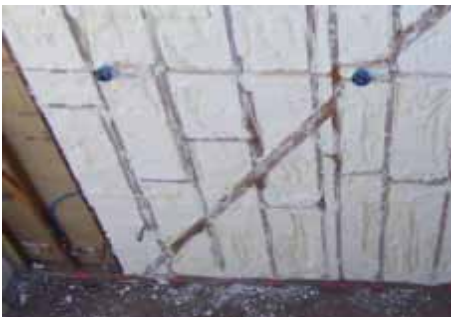
Fig. 9: Exposed wall framing
