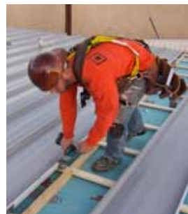
Fig. 14: Metal roof installation
