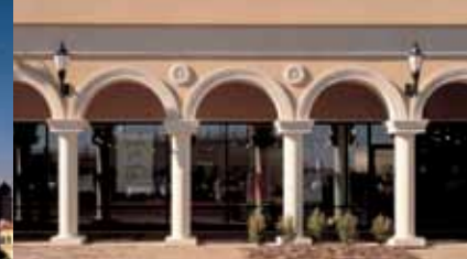
San Marcos Mall San Marcos, TX
