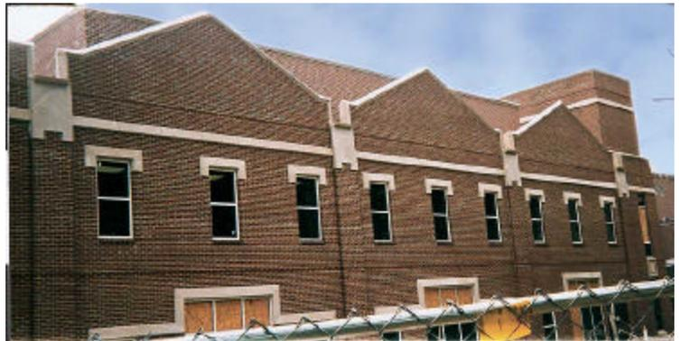
In 1873, HVAC screen walls were not needed because there wasn't a whole lot of equipment that needed to be located on the roof of a building. When new HVAC equipment was installed on the roof of the First Annex, however, the contractor was asked to hide it from view. Further, he was told that such a screen wall needed to both match the building's brick exterior perfectly AND be light enough to be placed on the roof.
