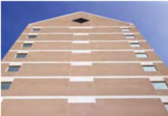
“Dryvit was selected because the ease of panelization of the Dryvit system helped solve the scheduling and weather challenges this project presented,” said Dryvit’s distributor Anne Lutz of the Lutz Company. According to Anne, approximately 120,000 square feet of Outsulation was used to build the 1,500 panels. The project, which started in November 2001, was completed in July 2002.
