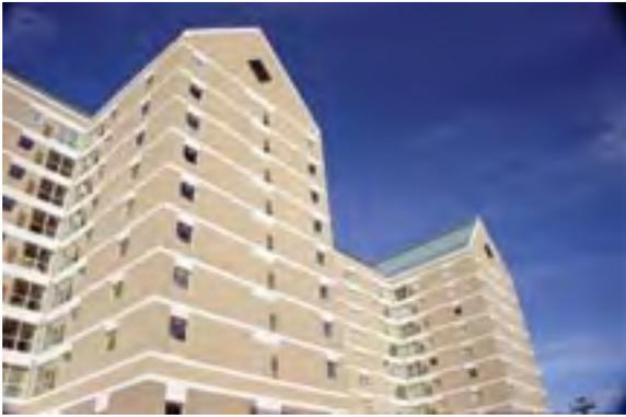
The Outsulite panel system is a lightweight (8psf), fully insulated prefabricated panel utilizing light gauge steel framing. A sheathing is installed to the framing, and then the air/ water resistive barrier, EPS (expanded polystyrene), reinforced base coat and finish coat follows.
