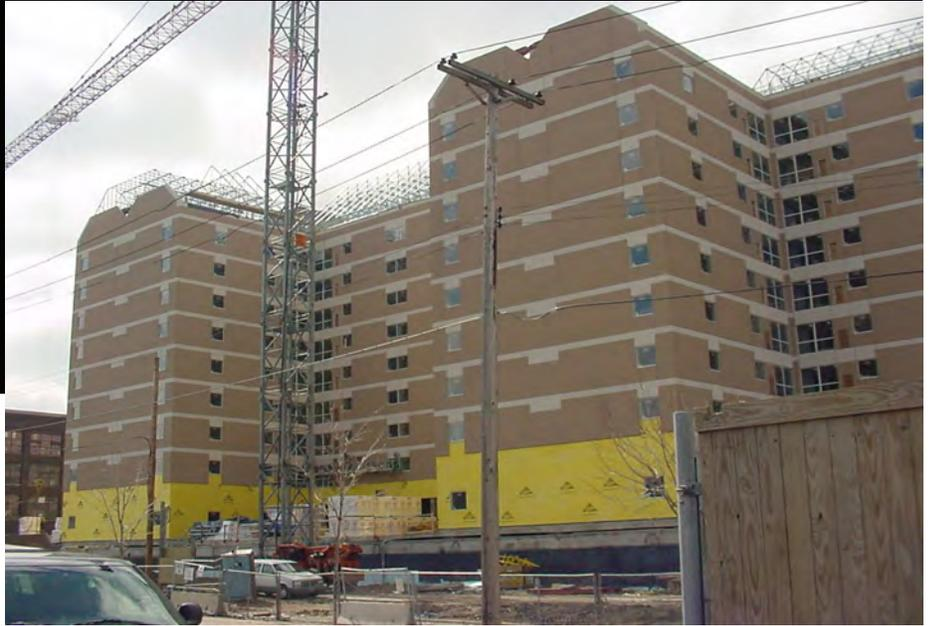
1,500 panels were hung, drying in the building, so interior work could begin.
