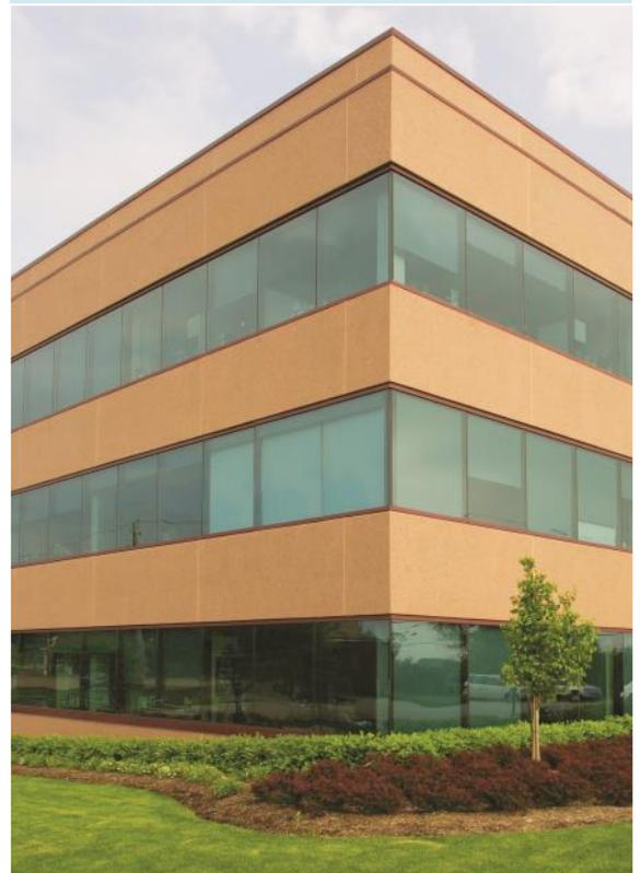
The Outsulation® Plus MD system was applied directly over the existing slate façade, providing continuous insulation and an air- and water-resistive barrier.
