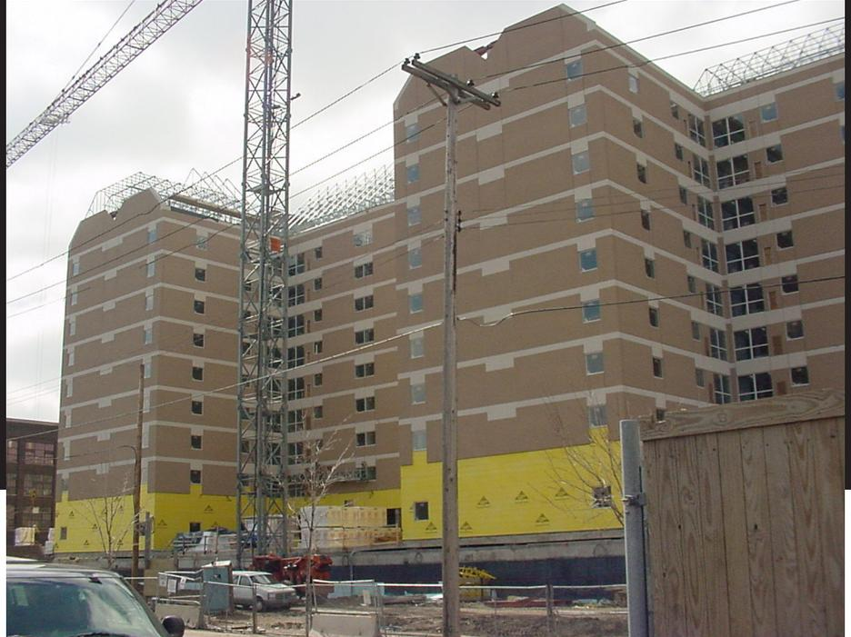
**1,500 panels were hung, drying in the building, so interior work could begin.**
