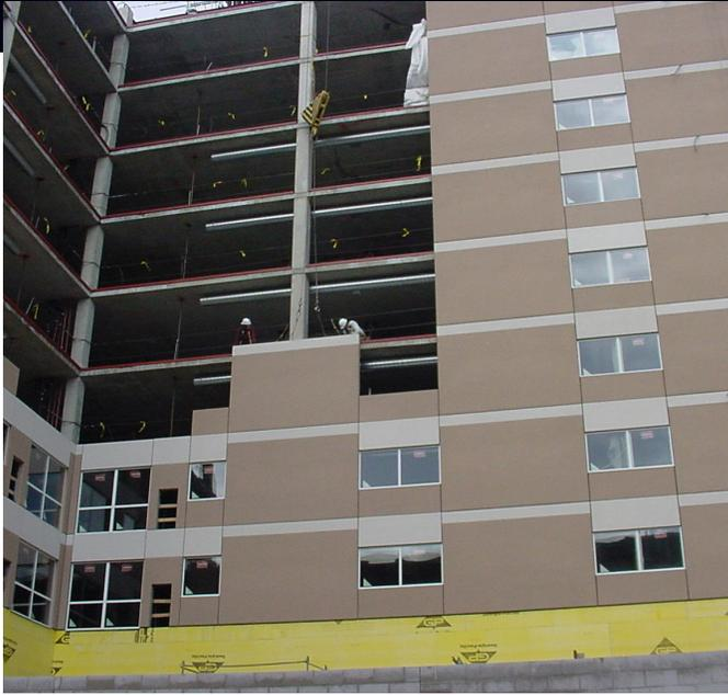
The Outsulite panel system is a lightweight (8psf), fully insulated prefabricated panel utilizing light gauge steel framing. A sheathing is installed to the framing, and then the air/ water resistive barrier, EPS (expanded polystyrene), reinforced base coat and finish coat follows.
