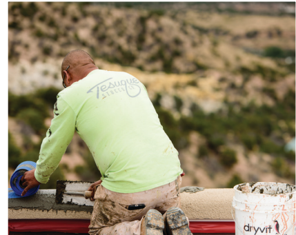
parapet repair
