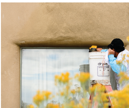
efflorescence removal
