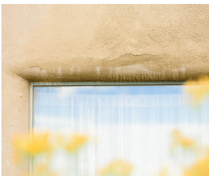
efflorescence
