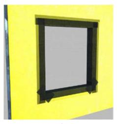
7) Allow material to set for approximately 15 minutes then apply a second liberal coat of AquaFlash Liquid and smooth out to ensure a continuous film free of voids, pinholes, or other discontinuities.
