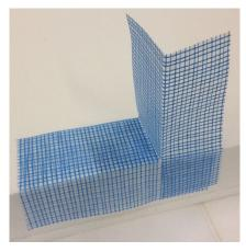
6) Install diagonal "butterflies" consisting of AquaFlash Liquid and AquaFlash Mesh at each sill/jamb corner – Figure 6.
