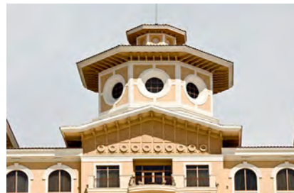
Shingle Creek Resort in Orlando, Fla. This massive resort property has numerous architectural features created by using EIFS. PHOTO COURTESY OF DRYVIT SYSTEMS INC.
