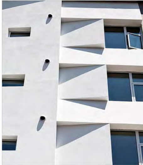
The Knickerbocker Commons project in Brooklyn, N.Y. features a façade insulation system with lotus effect technology developed by Sto Corp. PHOTO COURTESY OF STO CORP.
